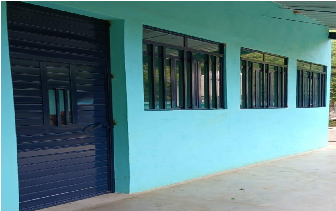
Completed Computer Lab Classroom
